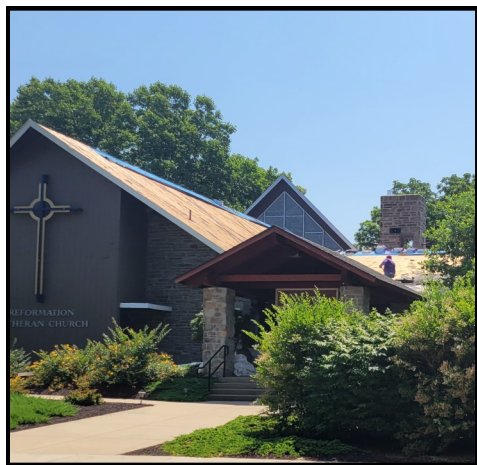
Roof work underway in June 2024.
