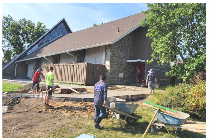
Major progress being made on the Reflection Garden project as shown on July 14.
