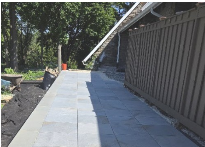
The patio is installed in the Reflection Garden.
